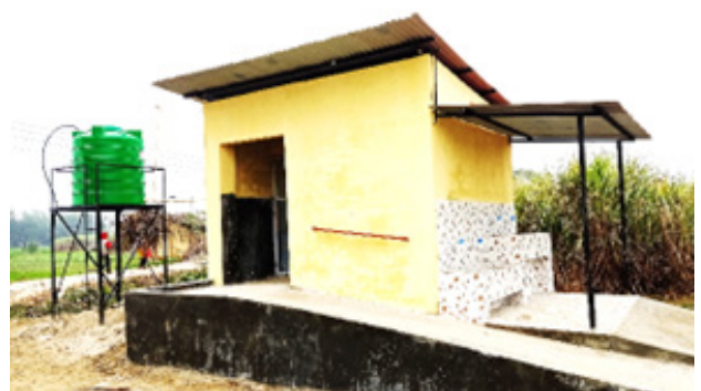
► Toilet constructed at Nepal Basic School, Badki Phulbariya, Devtal Municipality-01
