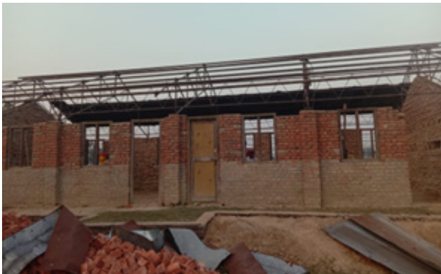
► Construction work completed at Achyut Basic School, Mahagadhimai Municipality-02, Bara
